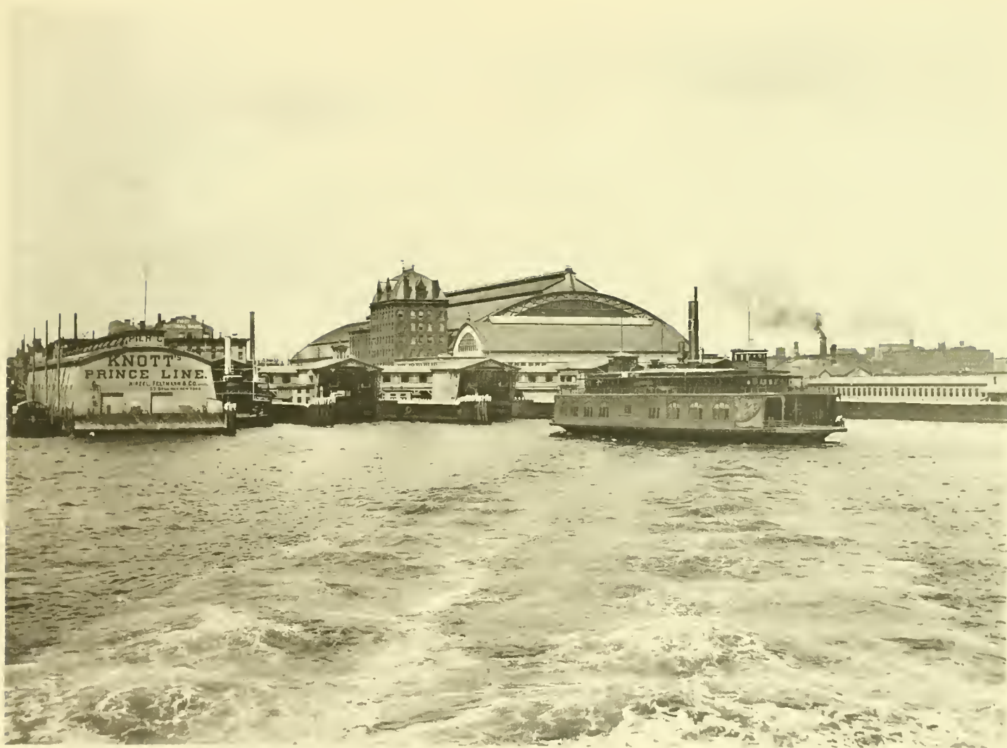
PENNSYLVANIA RAILROAD STATION—JERSEY CITY.
